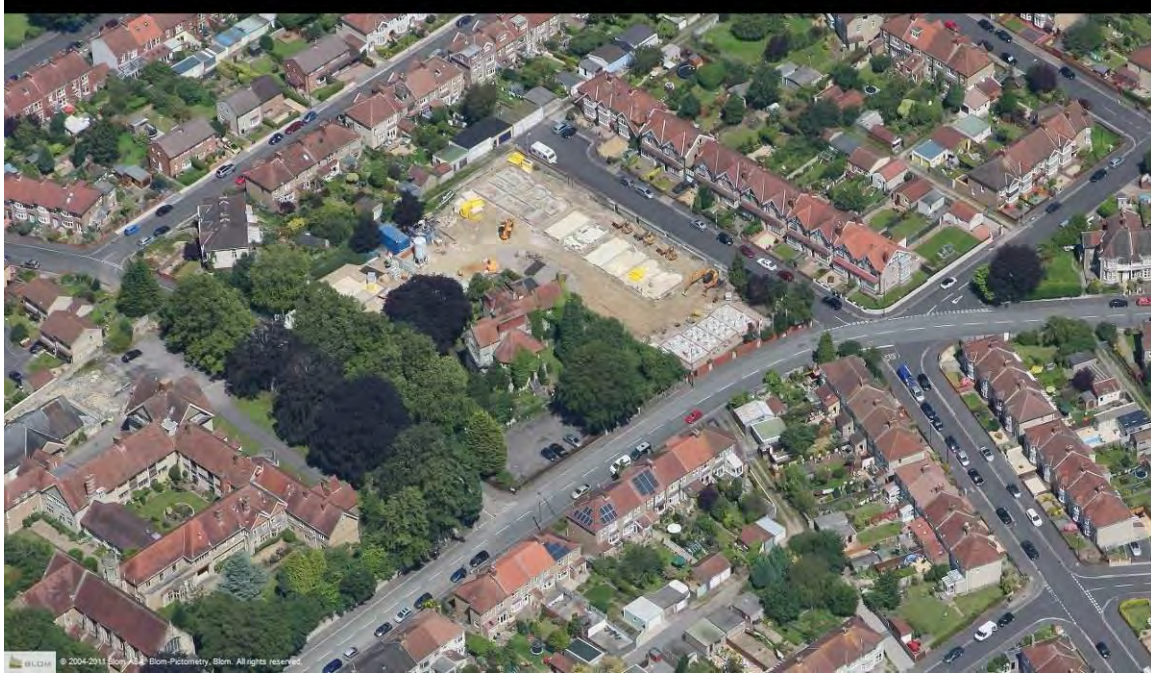
Aerial view of site looking north – note former St Peter's Hospice site under construction now complete and occupied. Footprint of new build properties can largely be seen.
